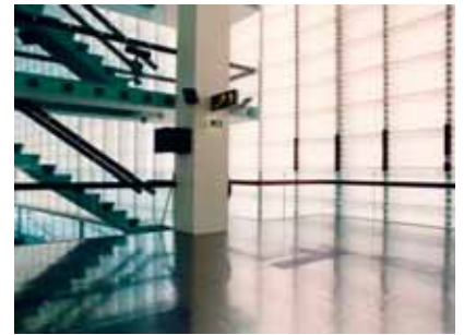
Lexan corrugated sheet system is used for the façade and the interior of the theater building in Rotterdam, Netherlands
