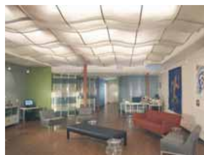
USG ceiling made from Lexan 90355 sheet
