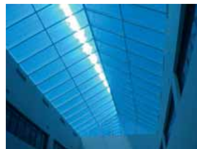
Both side UV protected Lexan Thermoclear Sun XP sheet is used for the roof glazing on this school in Al Wasel, UAE Dubai
