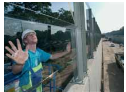
Soundscreen alongside the high speed railway line between The Netherlands and Antwerp from Koker Peerdobos
