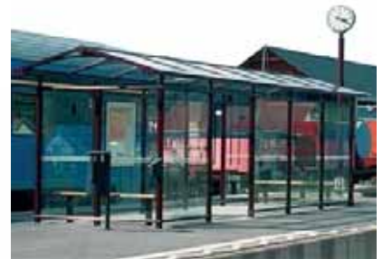
Lexan Margard* sheet is used for this train station shelter because of its high impact and abrasion resistance and durability for possible vandalism
