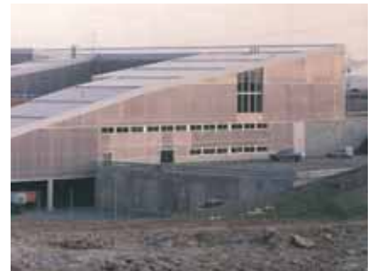
With its high light transmission and thermal insulation properties, Lexan Thermoclick* sheet was chosen by architect firm Abalos & Herreros for the vertical cladding of this building
